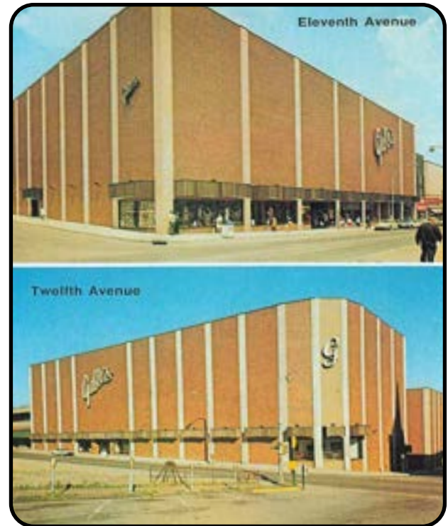
The modernized building without windows.
