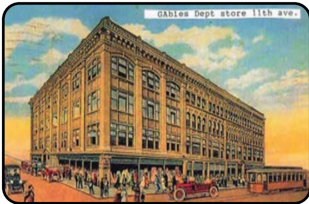
The original building with windows.
